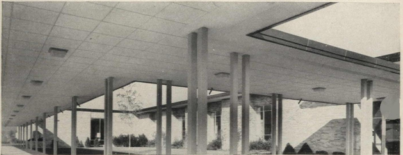
Elizabeth Seton High School, South Holland, Illinois used steel rustication strips on under side of canopy.
