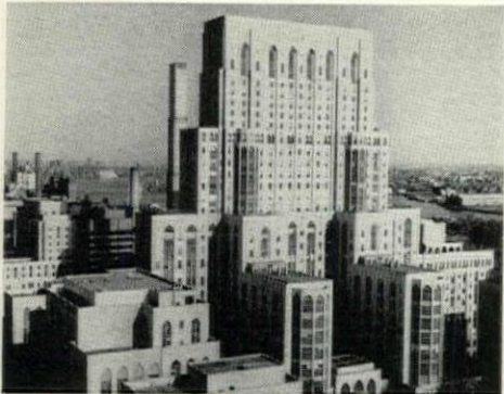
NEW YORK HOSPITAL- CORNELL MEDICAL COLLEGE ASSOCIATION BUILDINGS Five miles of Cheney Flashings installed in 1930
