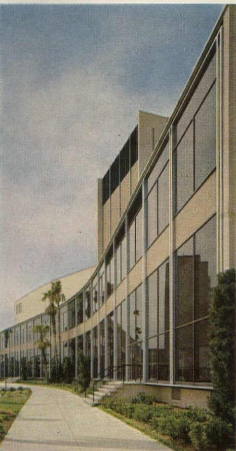
Civic Auditorium, Jacksonville, Florida. Architect: Kemp, Bunch & Jackson, Jacksonville.
