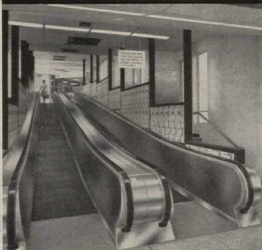
FOUR Montgomery POWER RAMPS at Stapleton have 40" tread width. Two Power Ramps have HORIZONTAL TRANSITION (horizontal entry — incline travel — horizontal exit.)
