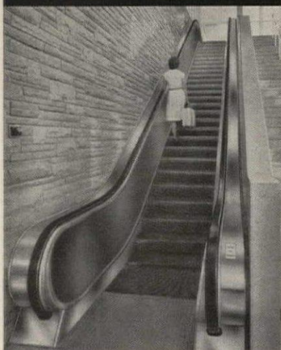
TEN Montgomery 48" ESCALATORS with exclusive feature of two-steps-level at entry and at exit move passengers rapidly and comfortably.
