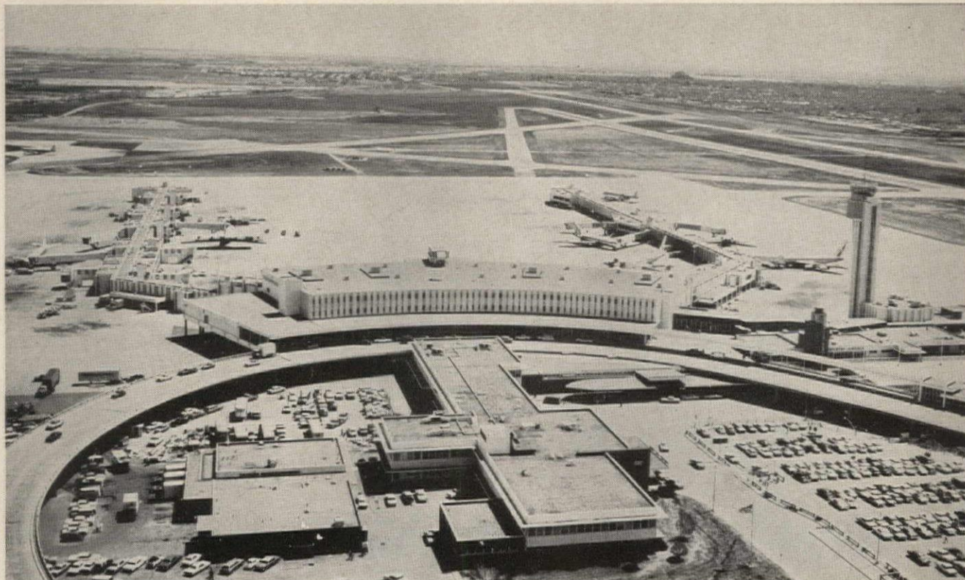
Montgomery provides Stapleton International Airport with every type of in-building transportation. More than 10,000 travelers use these facilities daily. Architect: PAUL R. REDDY / General Contractors: Olson Construction Co., Gerald Phipps, Inc., Hensel Phelps Construction Co.
