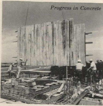
SYMONS STEEL-PLY FORMS GANGED AND LINED
