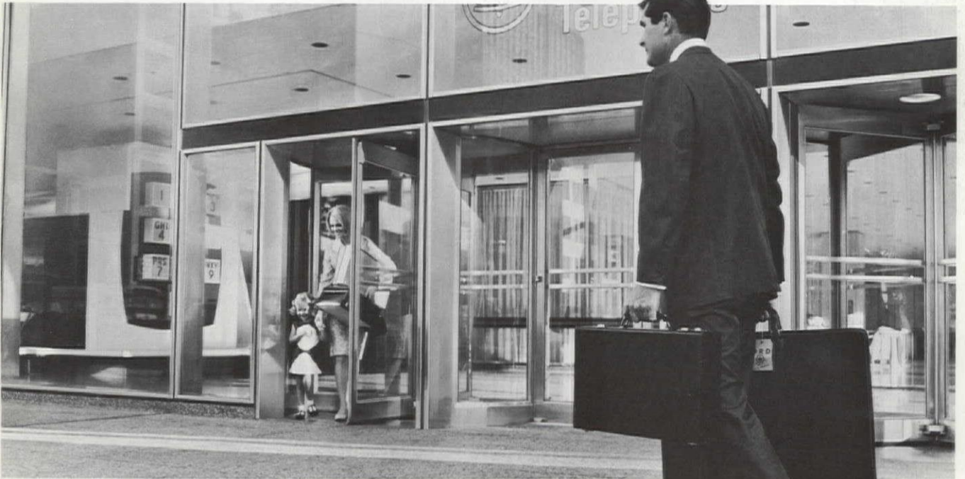
Door wings return to quarterline after each use. The entrance shown is one of 12 Revolvomatic doors extending an "open arms welcome" to the Chicago headquarters of Illinois Bell Telephone Company.
