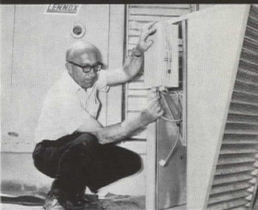
Simple "plug-in" connections for fresh air intake.
