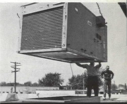
All-weather unit bolts to frame, needs no other sealing.
