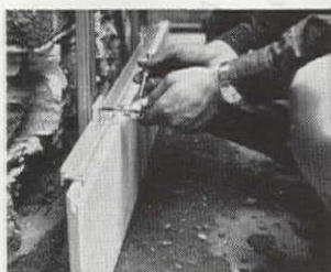
Horizontal members fastened by special clamps.
