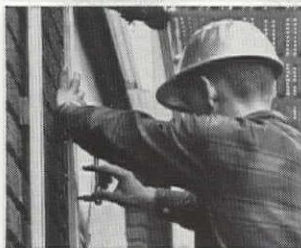
Vertical struts are anchored to existing facade.
