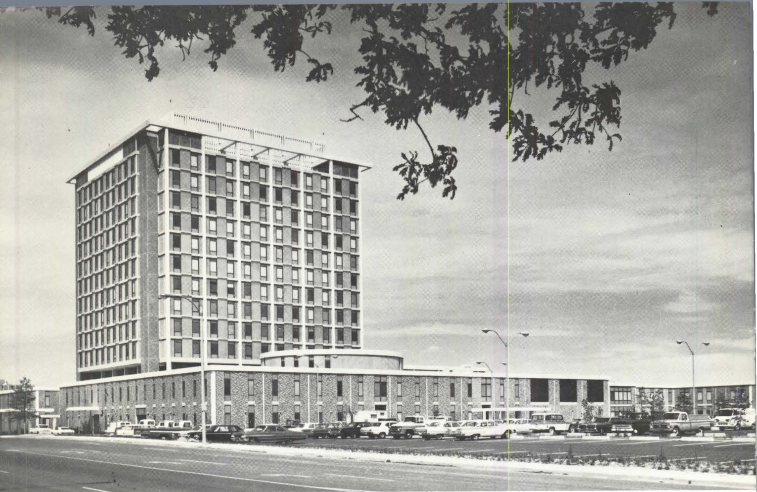
ABOVE—Veterans Administration Hospital, Memphis. Architects: A. L. Aydelott and Associates. General Contractor: Henry C. Beck Co. Seven Dover Gearless Elevators with Computamatic group supervisory control; 4000/5000 lbs. capacities; 500 FPM. Three Dover Oildraulic Elevators; 5000/6000 lbs. capacities; 60 FPM. Installed by Dover Elevator Co.
