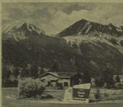
Information Center, Cape Perpetua, Oregon, above, and Ranger Station, Inyo National Forest, California, are compatible additions to our parks.
