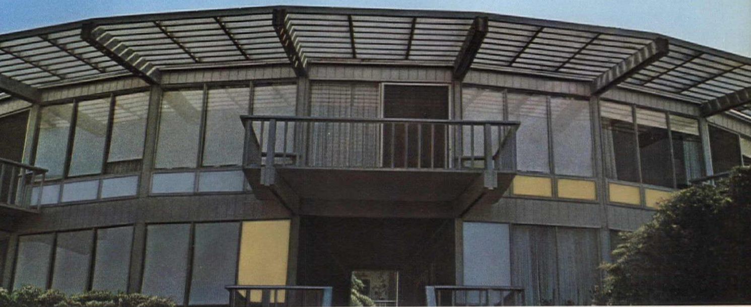
GLASWELD INSTALLED APRIL 1960, PHOTO TAKEN JUNE 1968.
