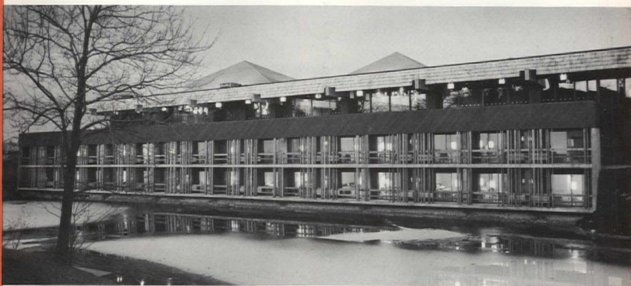
Sheraton-Wayfarer Convention Center in Bedford, N.H. is built into the bank of a brook.
