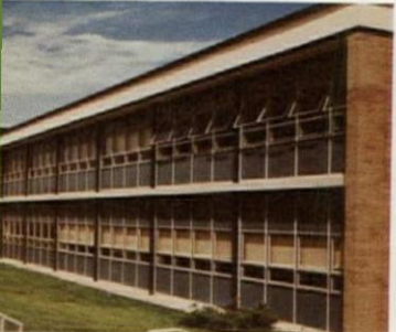
St. Croix School - Omaha, Nebraska Architect - Martin, Money and Assoc. Contractor - Butler Construction Co.
