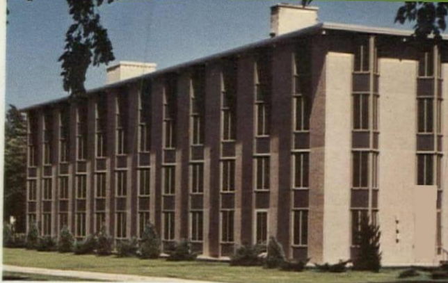
Dormitory for Duchesne College - Omaha, Nebraska Architect - Leo A. Daly Contractor - Butler Const. Co.
