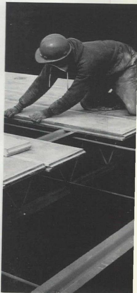
Steel-edged gypsum planks are welded to steel bar joists and to each other.
