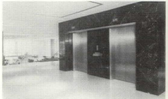
Express service to upper floors is provided by two high speed Montgomery elevators.
