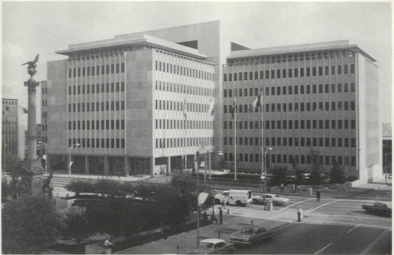
Caterpillar Administration Building and Employees Parking Garage, Peoria, Illinois. Architect: Smith, Smith, Haines, Lundberg & Wæhler; New York. Contractor: Huber, Hunt & Nichols, Inc.; Indianapolis.
