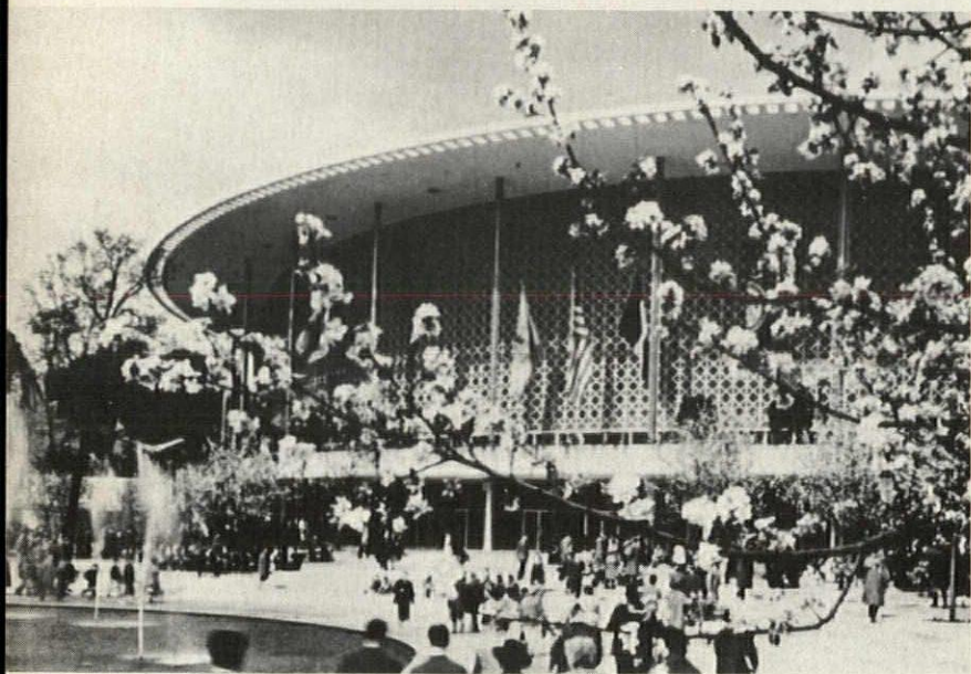
American National Exhibition, Moscow, with reinforced plastic roof and columns. Architects: George Nelson & Co., Inc. US Pavilion, Brussels World's Fair, with reinforced plastic roof, acrylic plastic walls. Architects: Edward Durell Stone & Associates.
