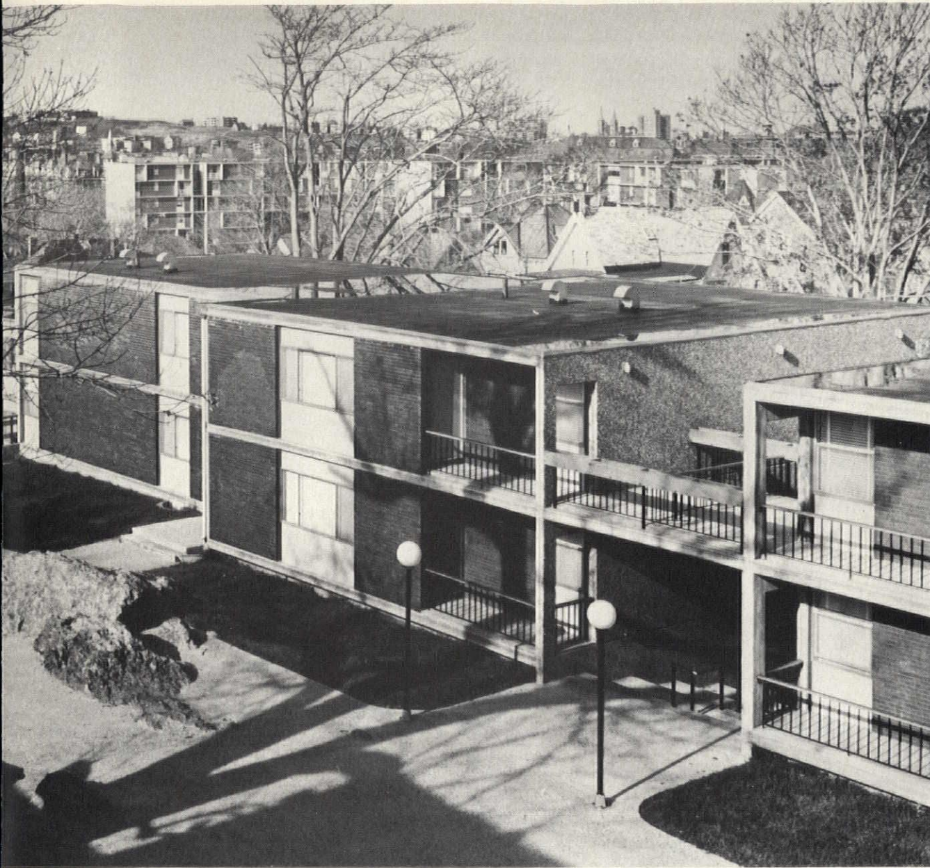
An early Techcrete project built in the Roxbury section of Boston and two under construction in Maine: both housing for the aging.
