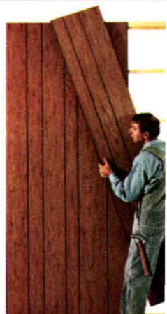
The One-Man Paneling. One man can panel a room by himself with 16"-wide Marlite PL
