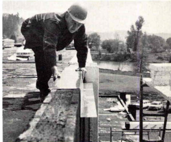
Pre-formed flashings were easily positioned prior to joining.
