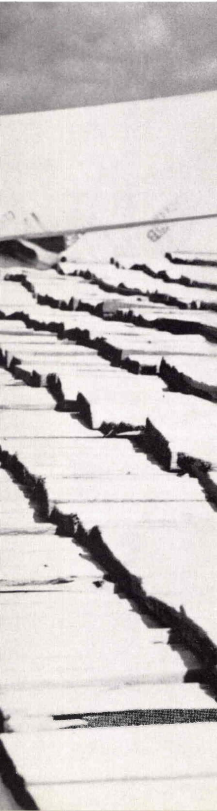
Pre-formed parts of Type 304, 26 gauge JalTEX stainless steel were delivered to the site by the mechanical contractor.
