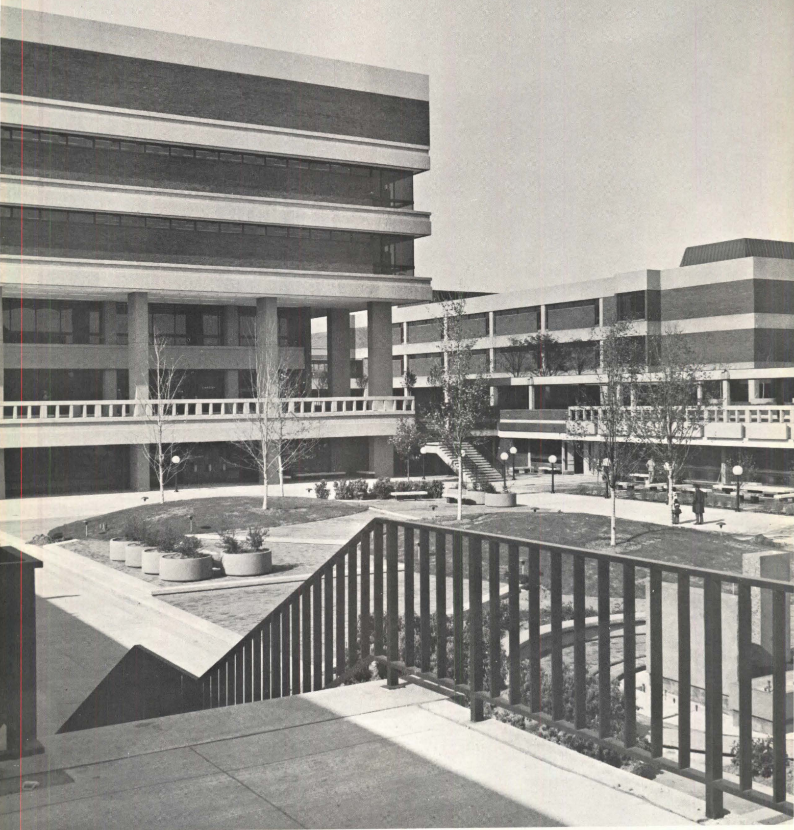
CUYAHOGA COMMUNITY COLLEGE, Cleveland, Ohio. Honor award winner in the 1970 Community and Junior College Design program. The complex was honored for "outstanding handling of a very limited site in an urban renewal area of the highly industrialized city of Cleveland." Architects: Outcalt-Rode-Kaplan-Curtis. General Contractor: Turner Construction Co. Twelve Dover Oilraulic and Electric elevators installed in seven buildings on the campus by Dover Elevator Co.
