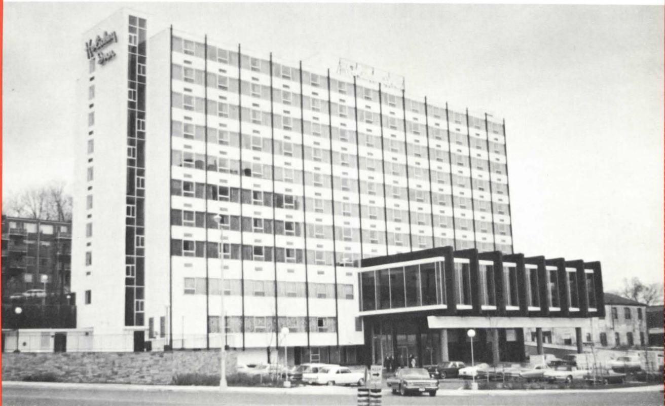
Vertical black anodized aluminum sections accent white brick exterior of the Holiday Inn at Rosslyn, Virginia.
