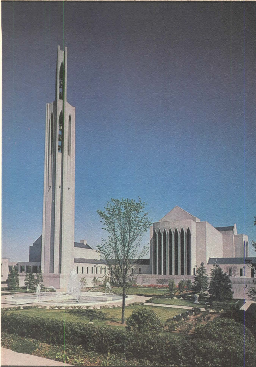
THE NATIONAL PRESBYTERIAN CHURCH AND CENTER, Washington, D. C., winner of the Building Stone Institute Award of Merit, Harold E. Wagoner & Associates, architects.
