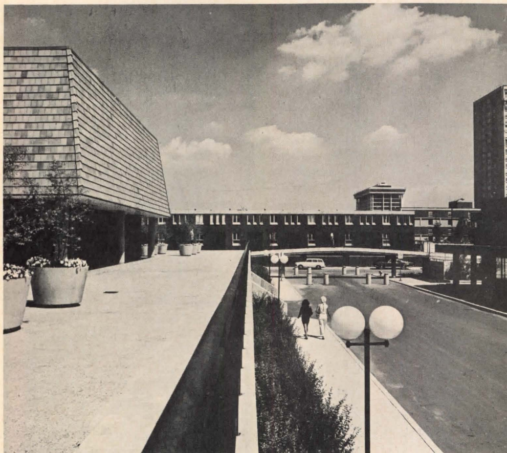
The terrace of the Community Center leads to the South Commons branch of the Drake Elementary School, seen in the background.
