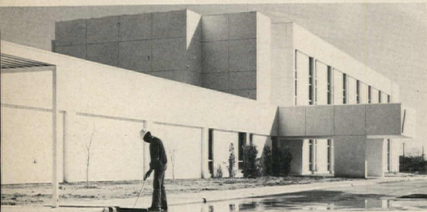
Baytown Hospital, Baytown, Texas, is built by Extendicare near a large industrial development complex now under construction for US Steel. The 189-bed, full-service facility, opened in February, was designed and built in 16 months. Golemon & Rolfe.
