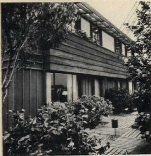
Modular duplex townhouse, shipped to its site by truck in four units, makes debut at NAHB convention. Frank Lloyd Wright Foundation is designer for National Homes.
