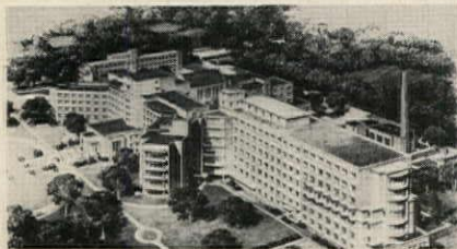
St. John's Hospital, Springfield, Missouri. Equipped with Security automatic cart handling system. Dumbwaiters by Otis.
