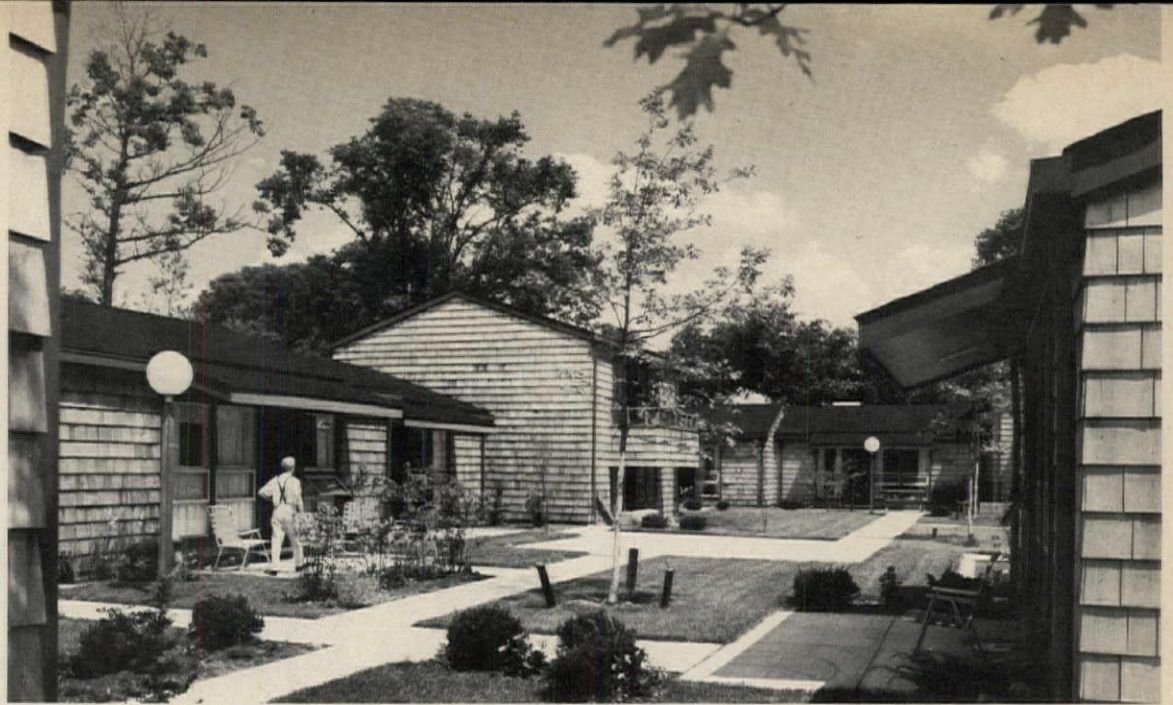
Good housing and a wholesome environment play major roles in prevention of illness and in keeping people happy. This includes dwellings for the elderly. The above shows a 40-unit low rent housing project for senior citizens in Wayne, Michigan. The units are oriented inward to the courtyards to invite sociability between the neighbors. The restricted sizes of the courtyards make gardening easy. William Kessler & Associates.
