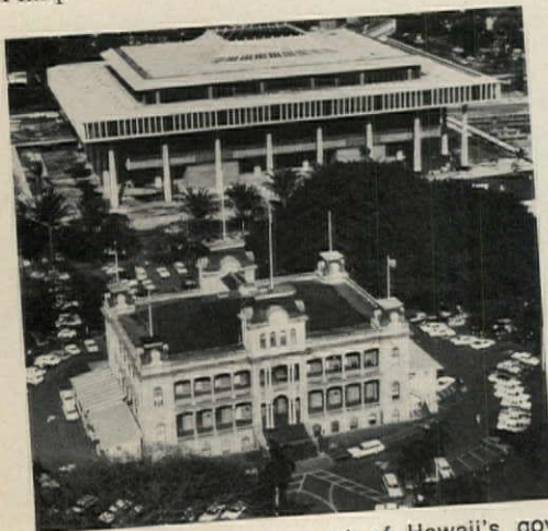
Behind Iolani Palace, seat of Hawaii's governments from 1882 until replaced, is the new capitol (John Carl Warnecke & Associates).
