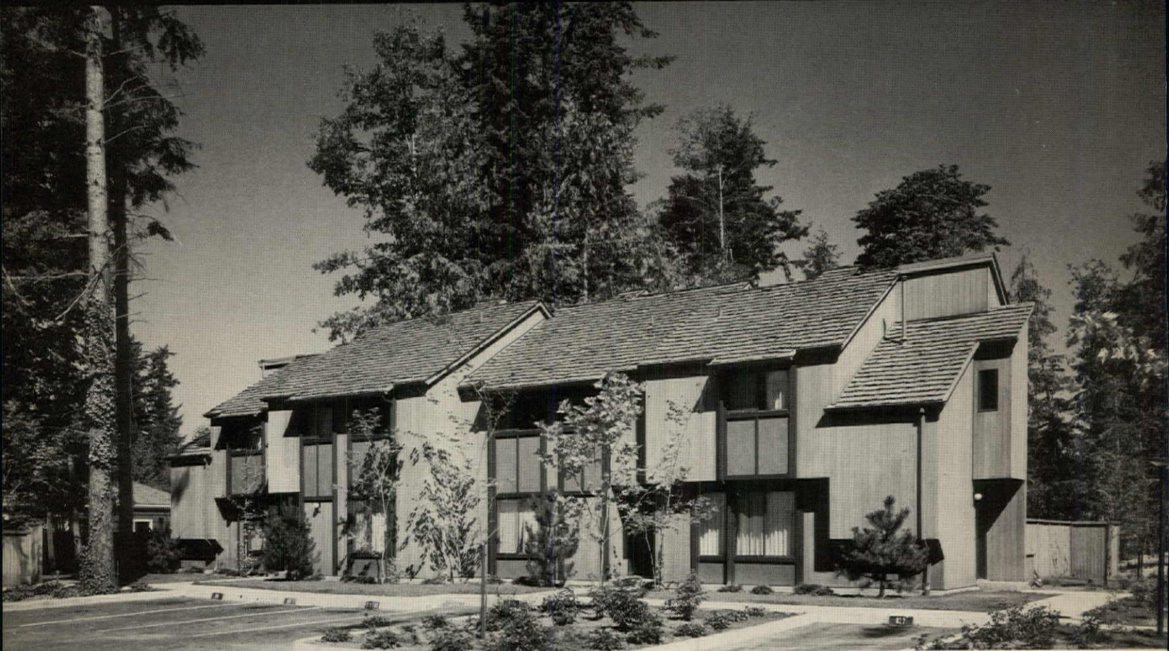
Turnkey Townhouses, Sedro Woolley, Washington. Certi-Split No. 1 Handsplit/Resawn Shakes, 24" x 3/4" to 1 1/4". Architects: Ron Thompson & Associates. Builder: Dujardin Construction.
