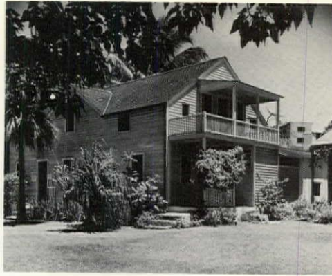
The erection of Yankee-styled prefabs posed problems, as the American Mission discovered when it wanted to erect a frame house with materials sent from Boston in 1820. When construction was delayed, frames were injured in the tropical sun, boards were lost and lumber was stolen. But the building was finally dedicated in 1833 and stands today as a historic landmark on King Street.
