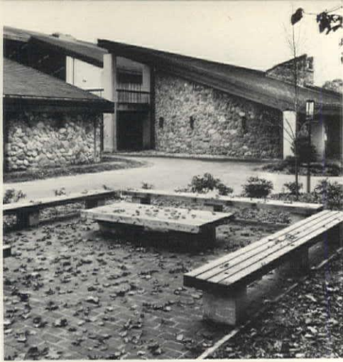
Two old horse barns house the administration offices and various academic activities and also inspire the design of new buildings at Brookdale Community College near Lincroft, New Jersey (The Shaver Partnership; The Office of B. Kellenyi, associated architects).
