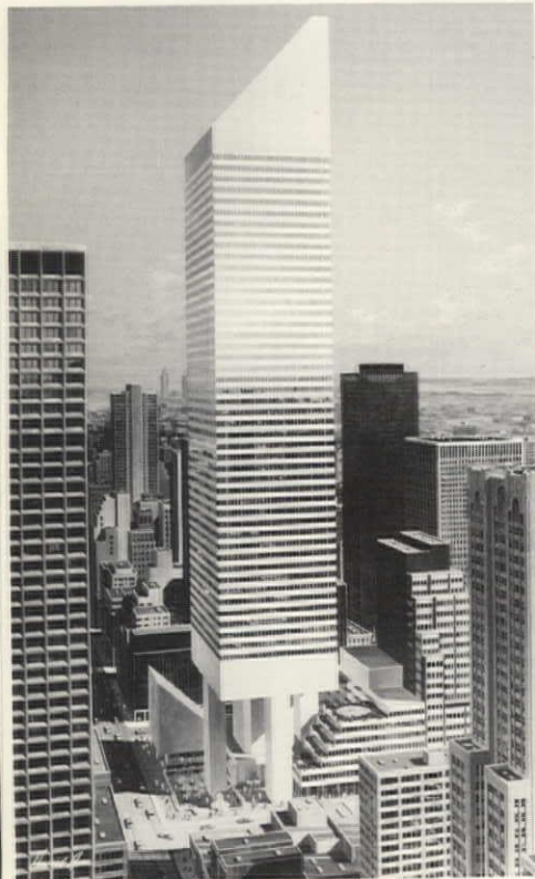
Steel frame of tower will be sheathed with reflective glass and aluminum bands.
