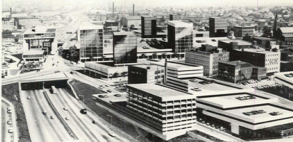
Precast concrete and reflective glass make up government center's exterior over freeway.
