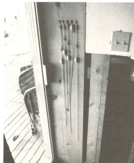
The controls for the solar-heated Davis house consist of strings to open and close dampers; there are no fans or thermostats.
