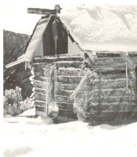
A reconstructed 1870 log cabin became a solar-heated guest house for the Allers family of Santa Fe in 1974. The southern facing roof slope accommodates 432 sq. ft. of solar collector to condition 650 sq. ft. of floor area.
