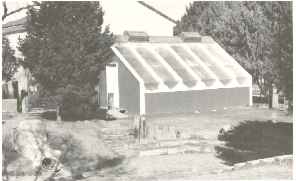
The "beadwall" of the Monte Vista Greenhouse is a direct and passive solar collector completely integrated in this facility for an experimental school program.
