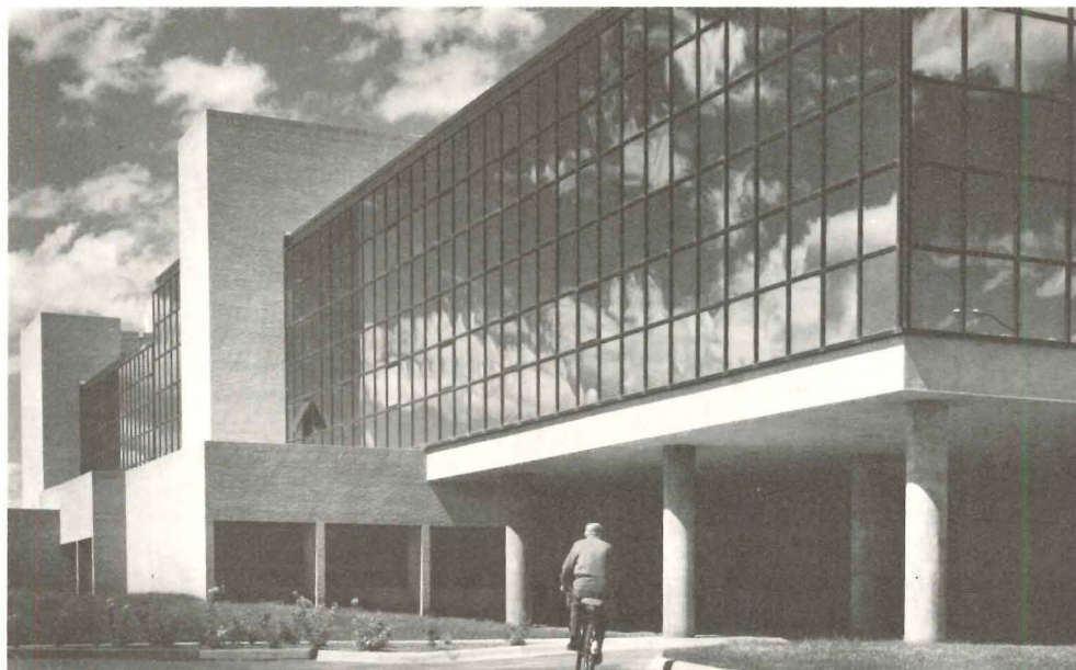
The Missoula, Montana, Community Hospital, designed by CTA.
