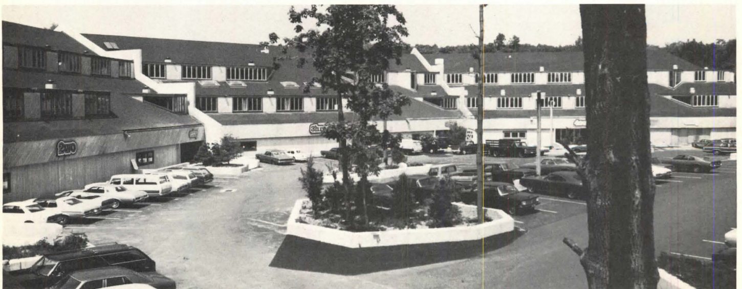
Sloping roof of The Exchange mall helps building appear small in scale despite its four levels and ¼-million square feet.
