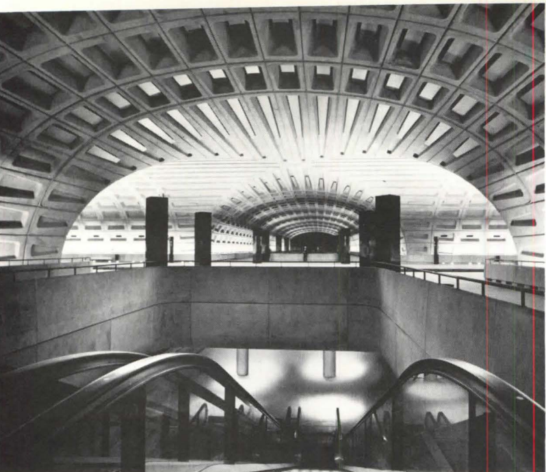
The mezzanines and escalators are free standing, at arm's length from the offered walls, their curved lines echoing the arc of the vault. The vertical elements above are pylons bearing signs.
