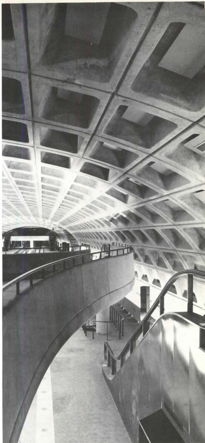
The mezzanines and escalators are free standing, at arm's length from the offered walls, their curved lines echoing the arc of the vault. The vertical elements above are pylons bearing signs.
