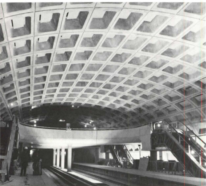
The mezzanines and escalators are free standing, at arm's length from the offered walls, their curved lines echoing the arc of the vault. The vertical elements above are pylons bearing signs.
