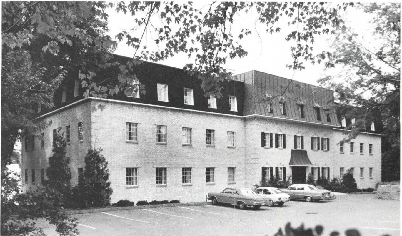
Mansard-roof facing and rearward sloping terrain make this new office condominium appear lower than its actual four stories.
