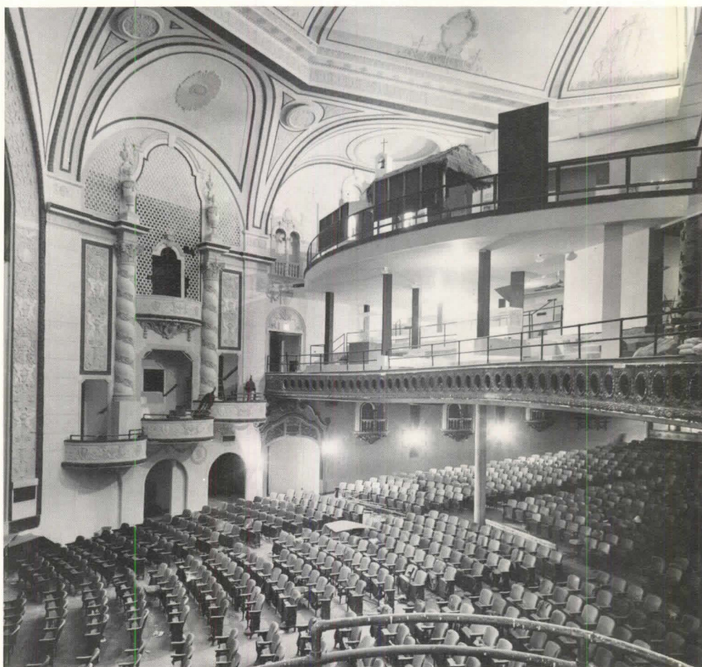
Three Hardy Holzman Pfeiffer recyclings: The Bronx's Cultural Ethnic Center, containing an experimental school, auditorium and offices, was a 1927 movie house.
