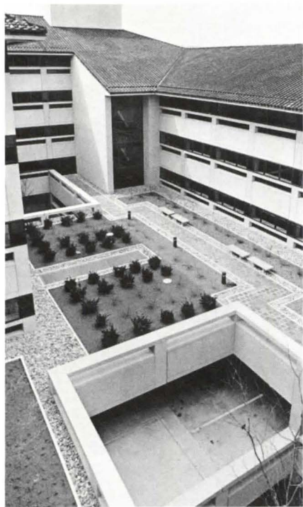
One of the sculptured courtyards that penetrate terraces to introduce natural light and air into garage areas.
