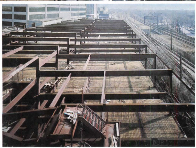
Parking deck structure.
