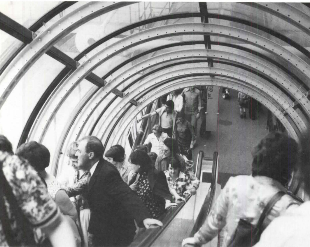
Escalator tubes during final construction phase (right) and in use (above).
