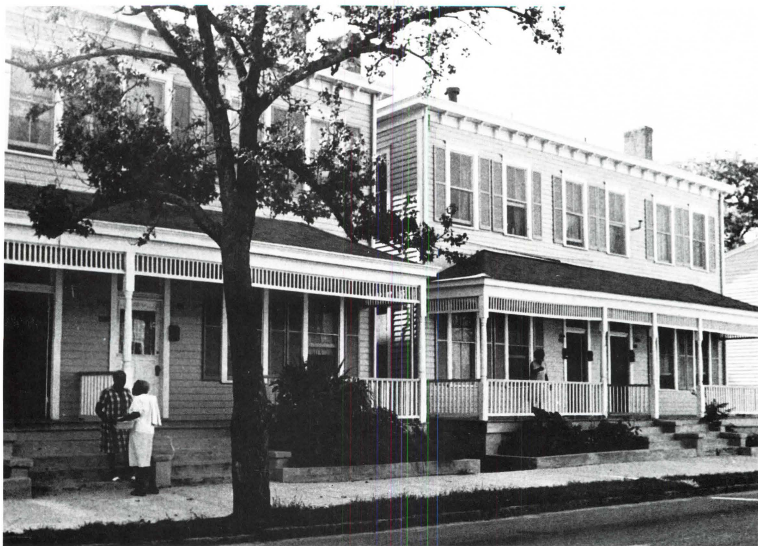
Across from the project on Price Street are privately rehabilitated homes; the hope is that others will follow.
