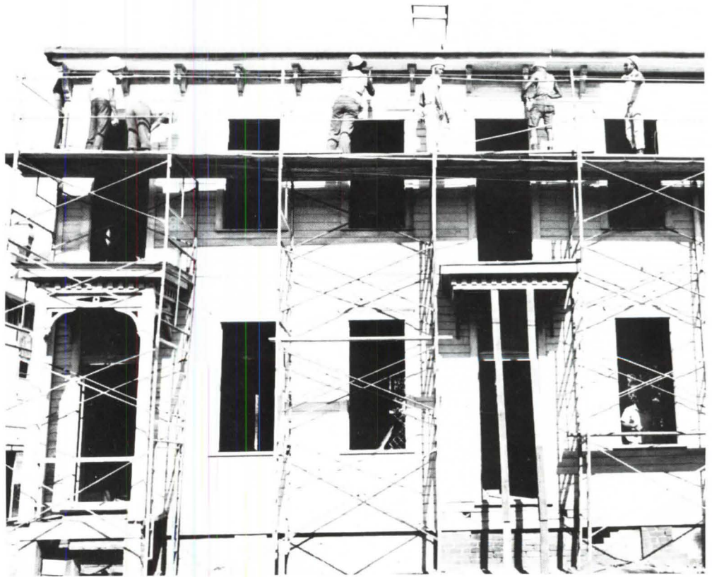
The area in early days was beyond city fire regulation zones and wood was used extensively; a row house on Price Street (bottom) is the first to be restored.
