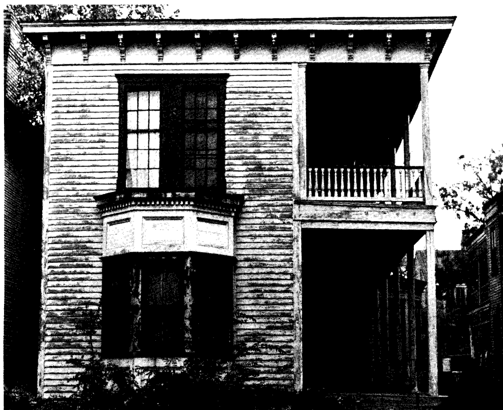
Added to the Register of Historic Places in 1974, the area's houses are 'carpenter Gothic,' trimmed with details bought from a building supply catalog.
