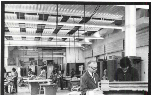
EFPs used for acoustic treatment at Burlington, Mass., High School Shop.
