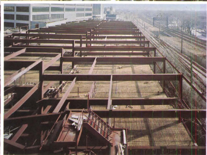
Parking deck structure.
