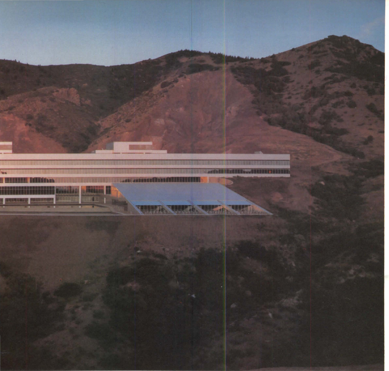
Ground level photos by Nick Wheeler
