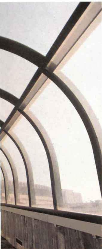
covered walkway at Yankee Stadium, New York City. LEXAN MR-4000's tough, ar-resistant coating makes it ideal for use in high-traffic applications.
