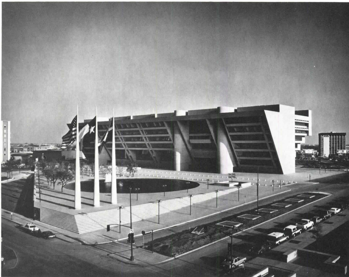
Park plaza, under which is space for 1,325 cars, extends 423 feet from the base of the cantilevered facade.
