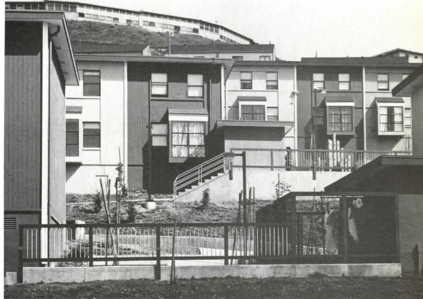
Formerly flat south facades (top) got bay windows on the lower floors; fences were upgraded.
