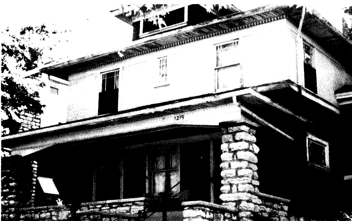
The Shirtwaist house, left, a Kansas City specialty, masonry below the belt and stucco or wood above. Across: a bird's-eye view of the Westport area.
