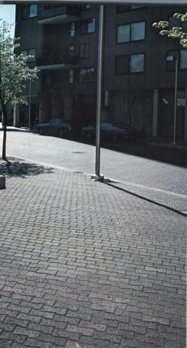
Roosevelt Island, New York City. This new town in the East River uses Concrete Pavers over a total area of 4½ acres for both pedestrian and vehicular traffic. Installation has been in use since 1972. Zion & Breen Associates, Landscape Architect & Site Planners.
