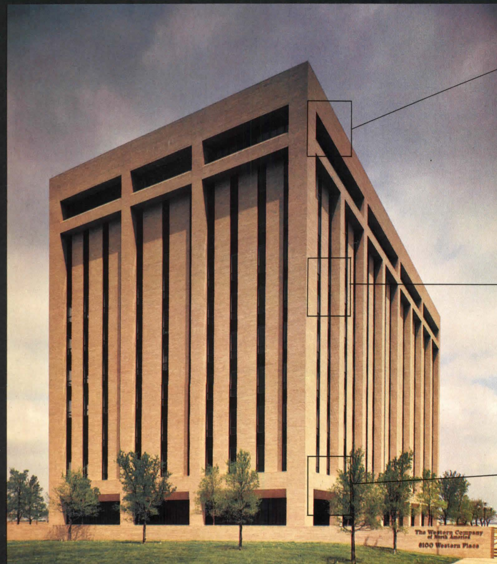
Hung soffit panels constructed of Acme Brick and high bond mortar produce deep, shadowed recesses below the parapet.
