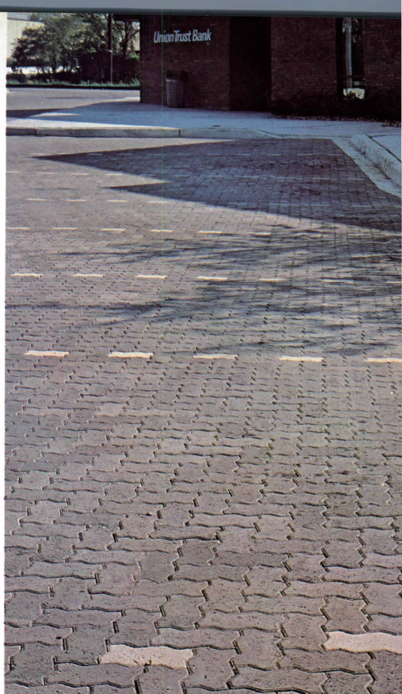
Parking area, Shopping Center, Baltimore, Maryland. Note that white units were installed to provide permanent parking space marking. Jewell Downing & Associates, Architects.
