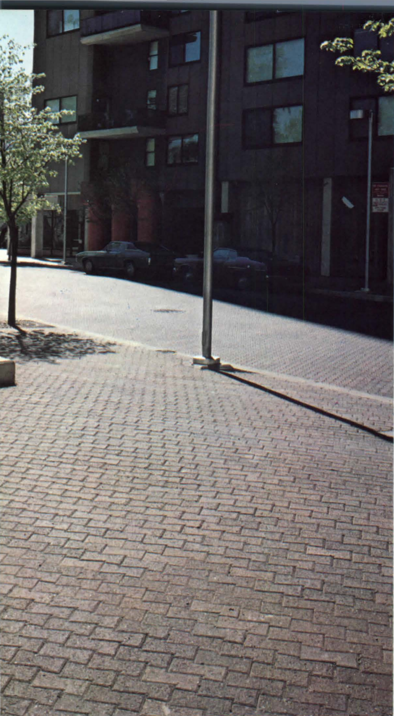
Roosevelt Island, New York City. This new town in the East River uses Concrete Pavers over a total area of 4 1/3 acres for both pedestrian and vehicular traffic. Installation has been in use since 1972. Zion & Breen Associates, Landscape Architect & Site Planners.
