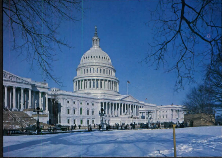
Capitol Building, Washington, D.C. / Arch: Architect of the Capitol
