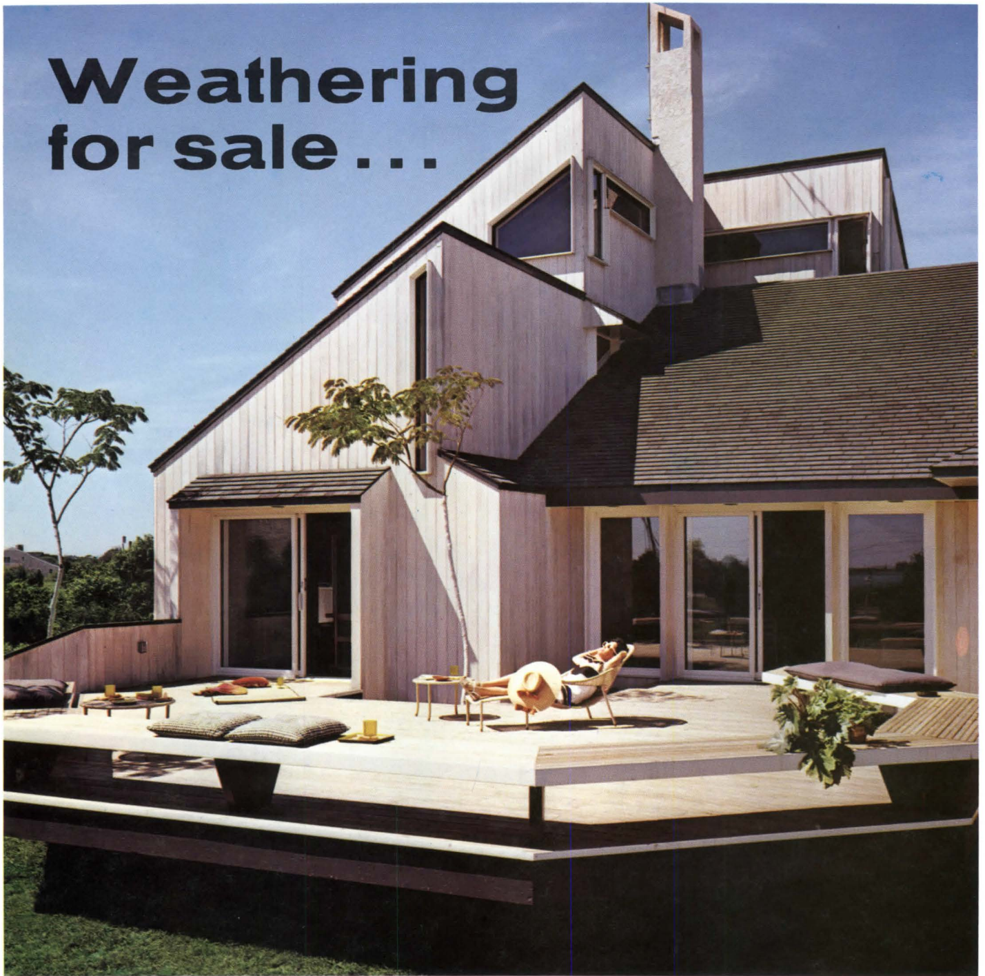
Long Island Home, Architect: Jay Lockett Sears, Quogue, Long Island; Wood surfaces treated with Cabot's #0241 Bleaching Oil for the weathered "driftwood" look.
