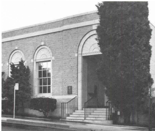
California Telephone & Telegraph Building Albany, New York, sealed with Thiokol polysulfide base sealant, 1947
