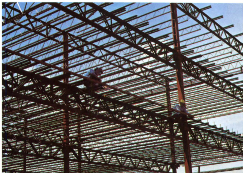
The simplicity and light weight of Vulcraft joists and joist girders make erection fast and easy.
