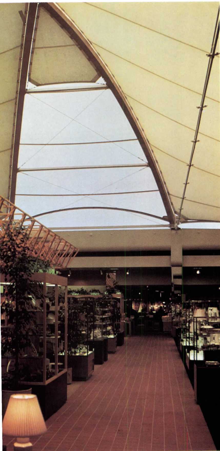
Above: Bullock's Department Store in San José, Cal. Note Grinnell Quick Response Sprinklers installed in a sprinkler line suspended from a cable below the fabric roof. Photo courtesy of Virgil R. Carter, Architect, Environmental Planning & Research, Inc.
