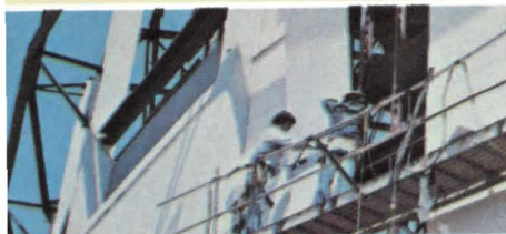
The J-M panels were face mounted to steel studding, requiring about 25 per cent less installation time than conventional masonry wall techniques.
