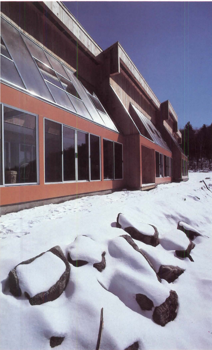
On the south (above and below) are three almost identical bays with rooms opening onto glazed solaria, which act as direct gain collectors. The north face (below right) has only narrow ventilation windows and a low sloping roof for wind protection.
