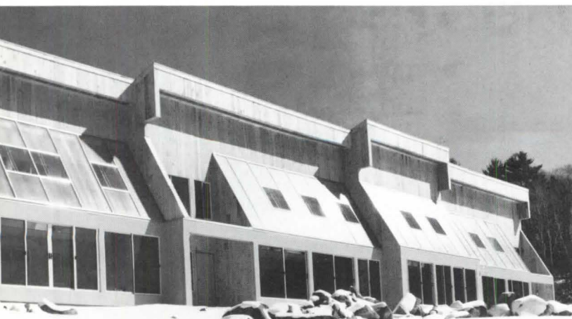
On the south (above and below) are three almost identical bays with rooms opening onto glazed solaria, which act as direct gain collectors. The north face (below right) has only narrow ventilation windows and a low sloping roof for wind protection.
