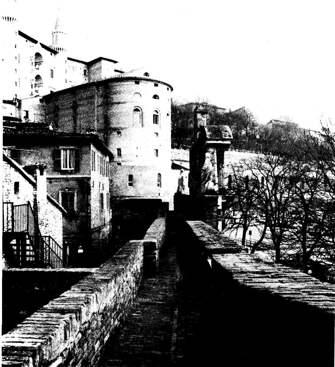
Across page, the ramp. The bottom photo shows its top level gallery, used for cultural and tourist activities. At left, a walkway on the city's wall leads to the rounded prow of the theater. Below, the theater's classical interior, under the renovation by de Carlo.
