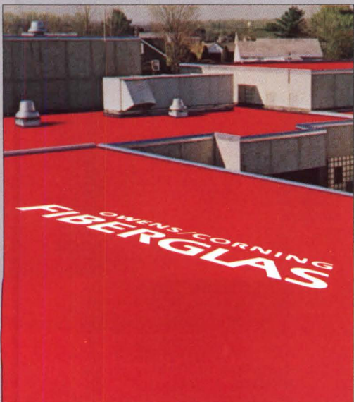
Double-layer Fiberglas insulation. New Perma Plus-2 system.† Gravel surface.
