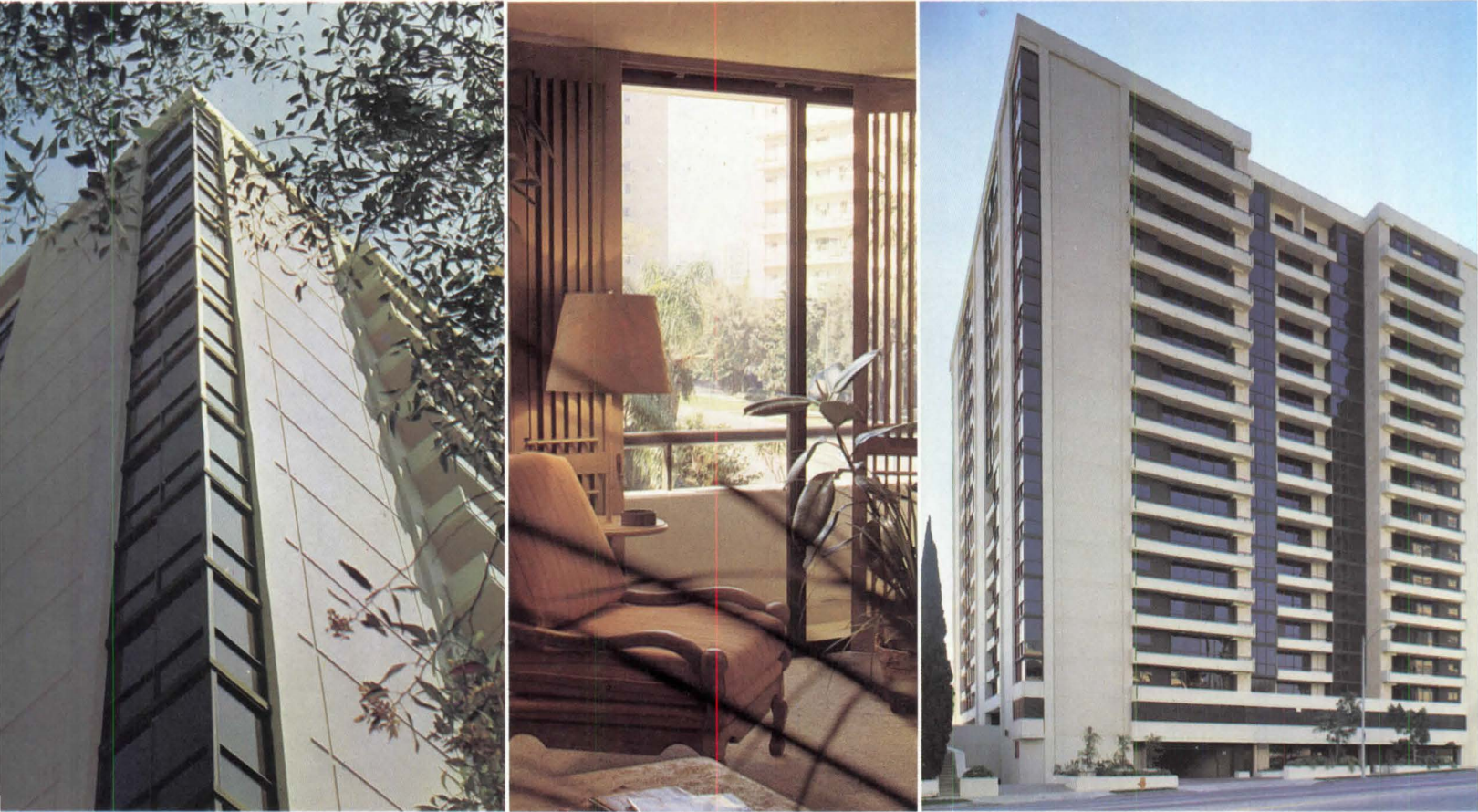
All glazing for this project handled by Fenestrol Corporation of Carson, California.
