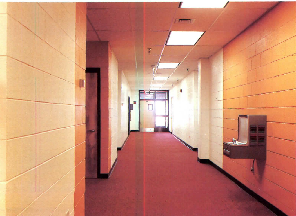
Interior walls of concrete masonry, used for thermal storage, are employed throughout the project.
