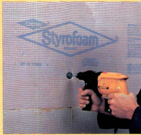
Fiberglass mesh is applied, mechanical anchors are attached
