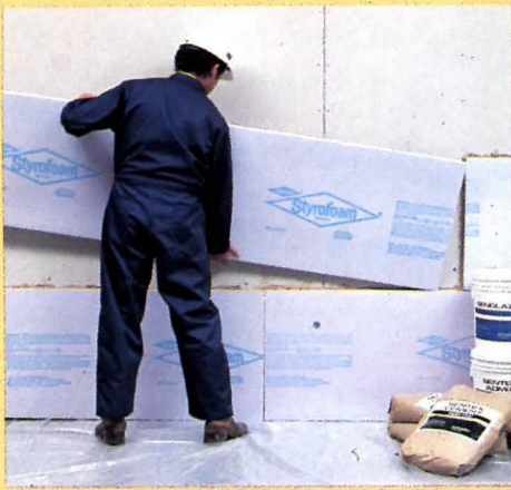
Boards of STYROFOAM brand insulation are set in place
