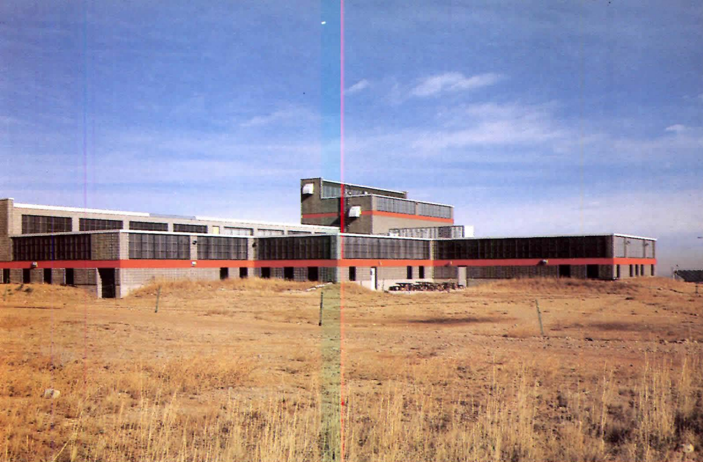
Concrete masonry Trombe walls are located behind the glazing which borders the upper portions of the building.
