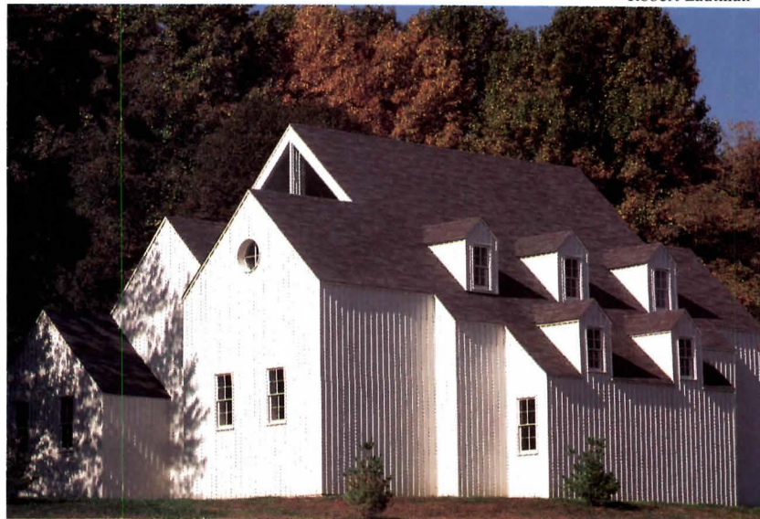
The addition's southwest corner, above, and sanctuary, top.
