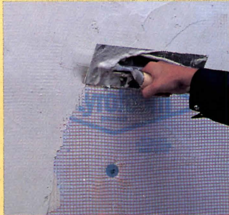
Base coat is applied with trowel
