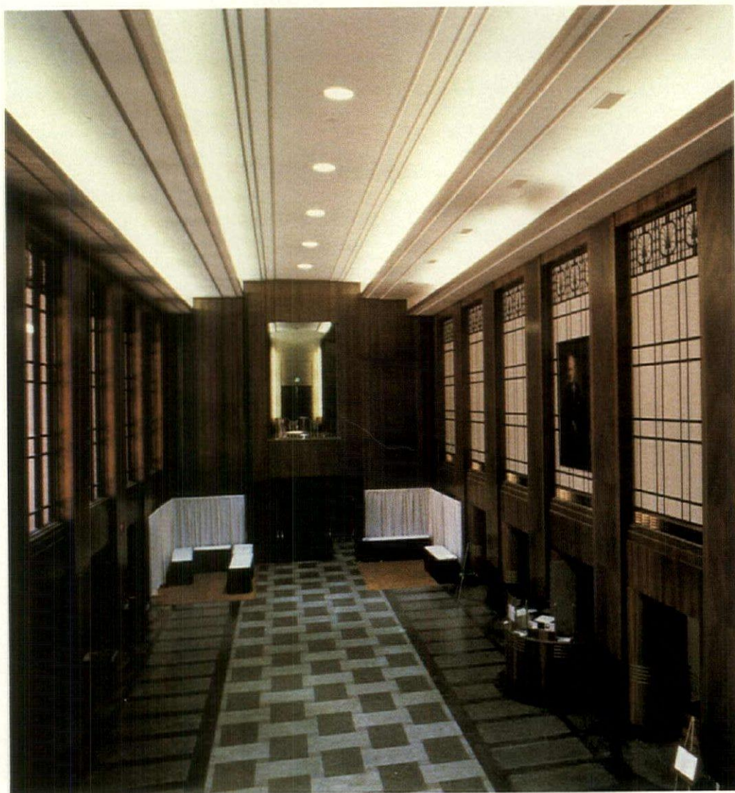
Cove lighting, restored with the help of old photographs, emphasizes clean lines of main lobby ceiling, once cluttered with surface-mounted fixtures.
