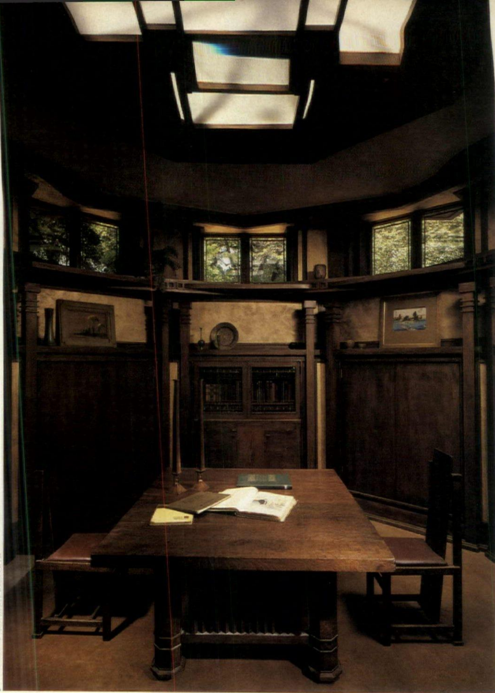
The octagonal library required a high light level for reading and presenting drawings to clients. In response to this need, Wright used a band of clerestory windows on seven of the eight sides, an 11-foot-diameter octagonal skylight that nearly covers the roof, and frosted glass panes set on a wooden framework. For relamping, the glass is simply pushed away.
