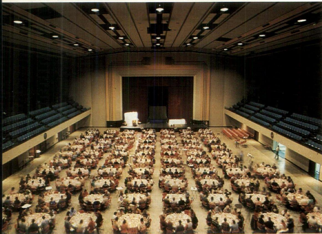
Multipurpose light ports in auditorium ceiling each hold five different fixtures.
