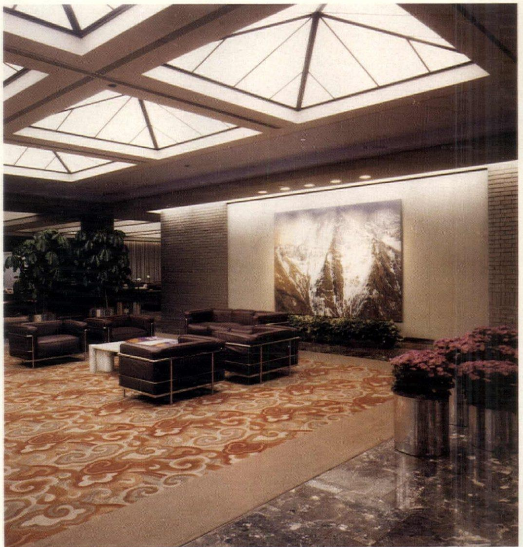
The main reception area (above and right) is highlighted with artificial skylight elements. To balance brightnesses, a continuous wall wash is used around the core wall. Highlighting is focused on a piece of art depicting a Rocky Mountain scene.
