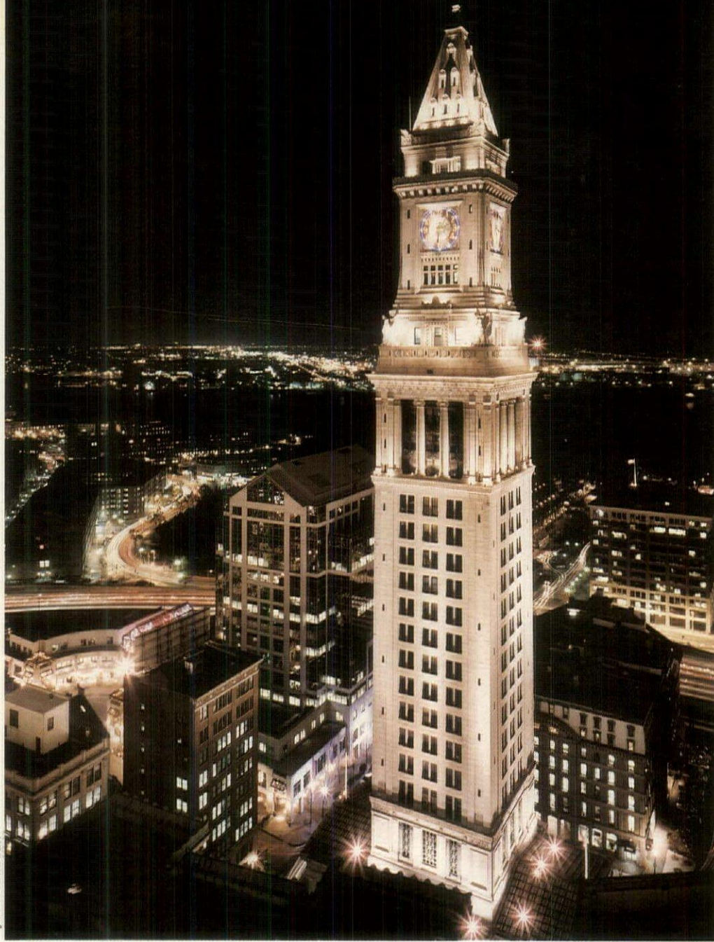
New lighting illuminates the Custom House from street to peak with the same amount of power previously used to light only the clock. Precisely focused PAR lamps light tower exterior.
