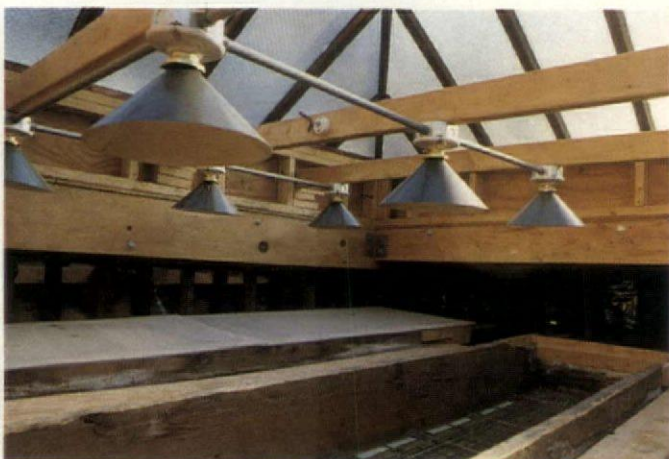
At night, electric lamps in the skylight wells replace daylight. These fixtures above the reception hall laylights are serviced via an access panel opening off the drafting room balcony. New thermal venting helps to disperse heat.
