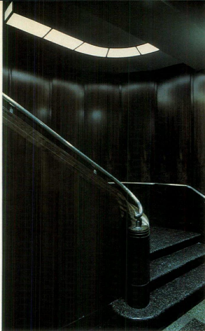
Refurbished linear fixture was converted from expensive incandescent to more economical fluorescent.
