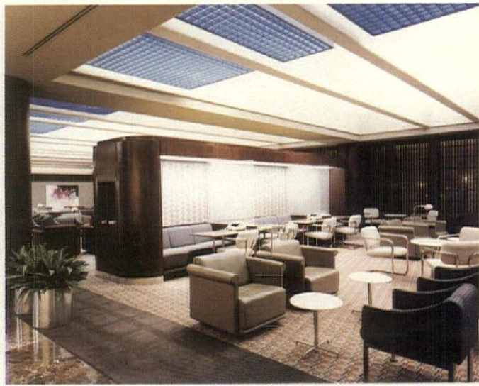
Banquettes have been fitted with miniature built-in luminous ceilings. These are illuminated with fluorescent strips, backlit by white acrylic panels fitted with louvers. The panels block the fluorescent strips from view.
