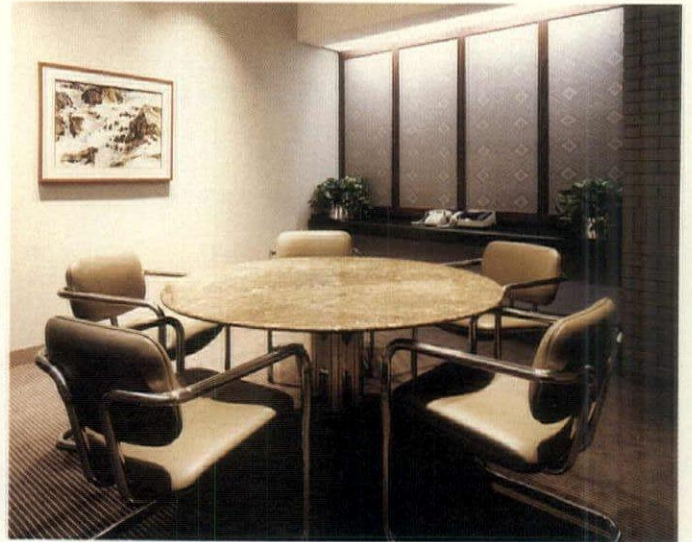
The fluorescent wall wash helps open the conference rooms visually. Incandescent accent luminaires are used to highlight artwork, and incandescent downlights provide task lighting at the table.
