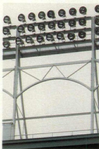
A black insert in each fixture lets photographers shoot at the lights from an angle without washing out the image.
