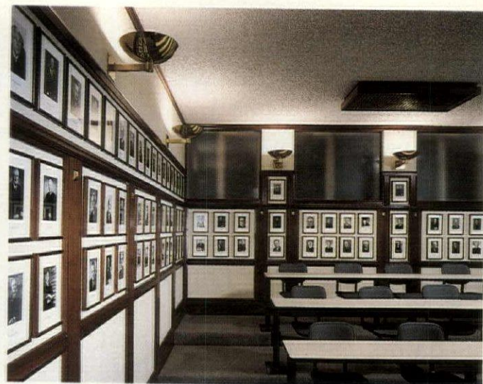
Brass-finished incandescent wall brackets provide soft uplighting for the alumni photo gallery lining the side and back walls of the classroom. Surface-mounted fluorescent luminaires with gold-colored louvers add general light for reading and note-taking.
