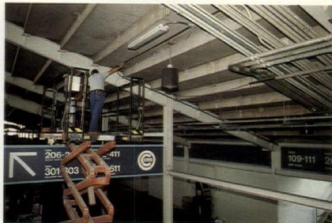
High pressure sodium was chosen to light the ramps and the concourse at the back of the seat deck because the back of the stadium is fairly open to the outside, where HPS sources are used in the parking lots and in the old-style street lamps with acorn style globes.
