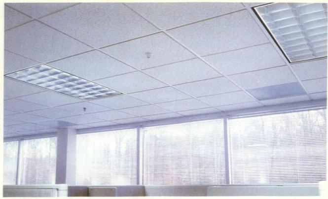
Figure 4A: Office with daylight compensation using dimming photo-sensor
