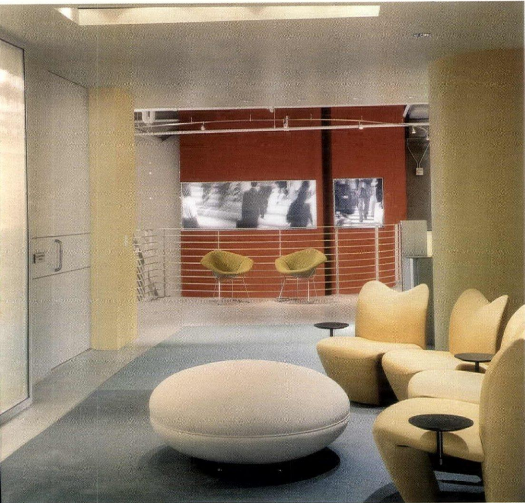
Above: A ceiling slot is equipped with low-voltage trackheads to illuminate an upstairs lounge area. In the background, tracklights on a curved monorail intensify the vivid red of a two-story wall and lend the reception area a feeling of brightness. Right: The office area where employees work primarily on computers, indirect pendants lamped with T5 fluorescent sources supply glare-free VDT illumination.
