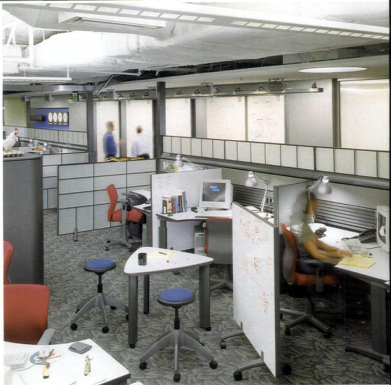
Above: A ceiling slot is equipped with low-voltage trackheads to illuminate an upstairs lounge area. In the background, tracklights on a curved monorail intensify the vivid red of a two-story wall and lend the reception area a feeling of brightness. Right: The office area where employees work primarily on computers, indirect pendants lamped with T5 fluorescent sources supply glare-free VDT illumination.
