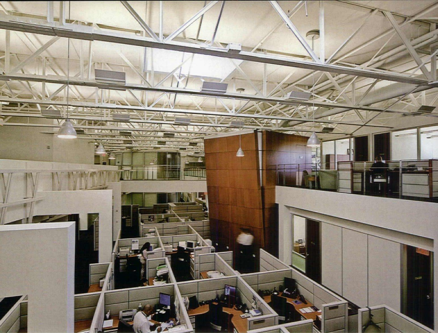
A standard control system and new fixtures were employed over the workspaces. A mix of recycled 100W ED17 metal halide and fluorescent sources were used on the mezzanine. Along the monumental staircase (facing page, left) recessed adjustable MR16s highlight the landing, while recessed slot fixtures provide both ambient illumination and a luminous design feature. In the 14th-floor conference room, recessed slot fixtures offer general illumination (facing page, bottom). Outside the 15th-floor conference room, a cove light and soffit linear fluorescents provide 20 footcandles (facing page, top).
