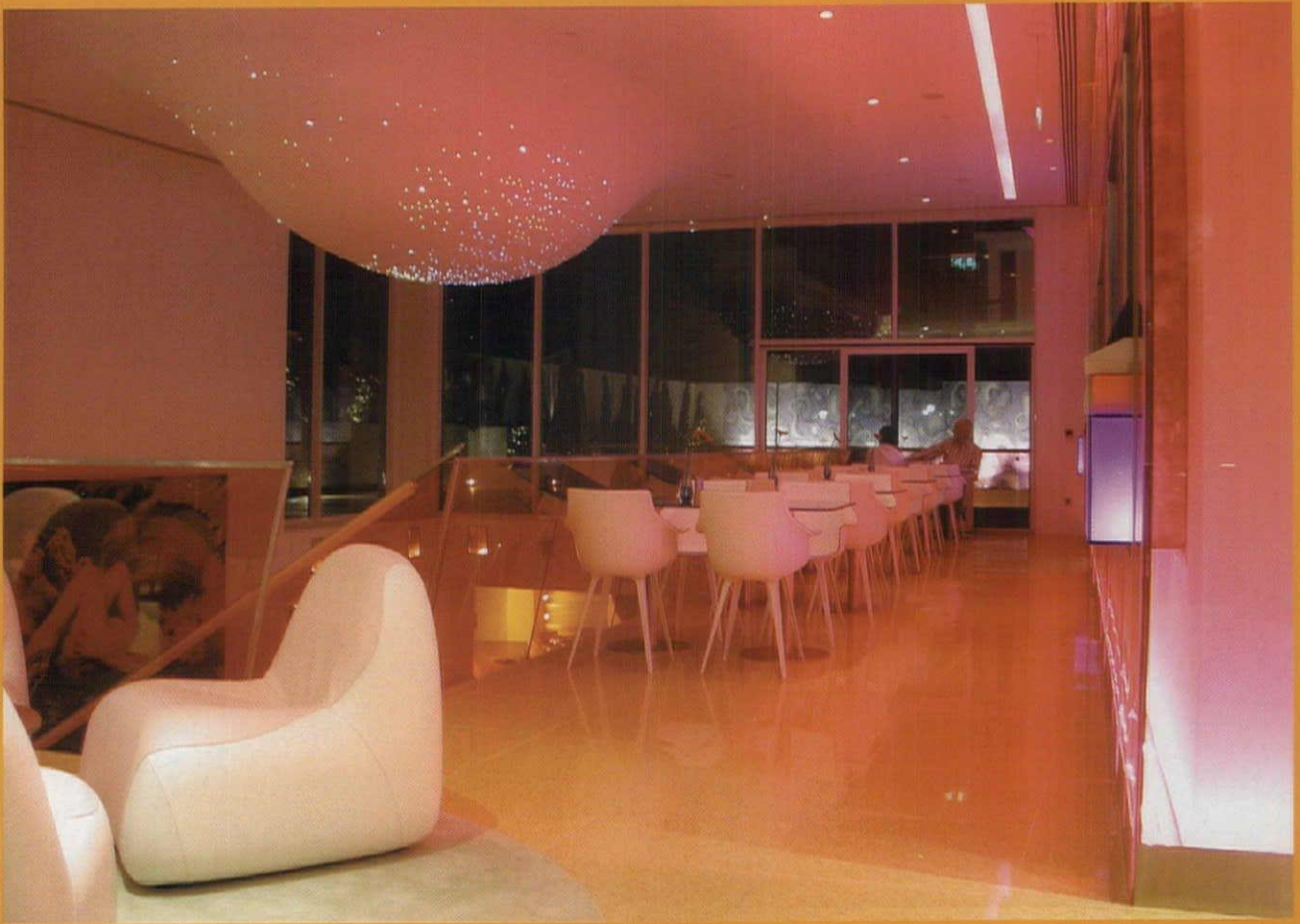
The curvaceous detail in the second-floor lounge ceiling is actually a luminaire, intended to look like "stars, with flickering lights." Fiber optic points are lit with an easily accessible metal halide source. Incandescent fixtures recessed in the wall uplight the disco-like ceiling element.
