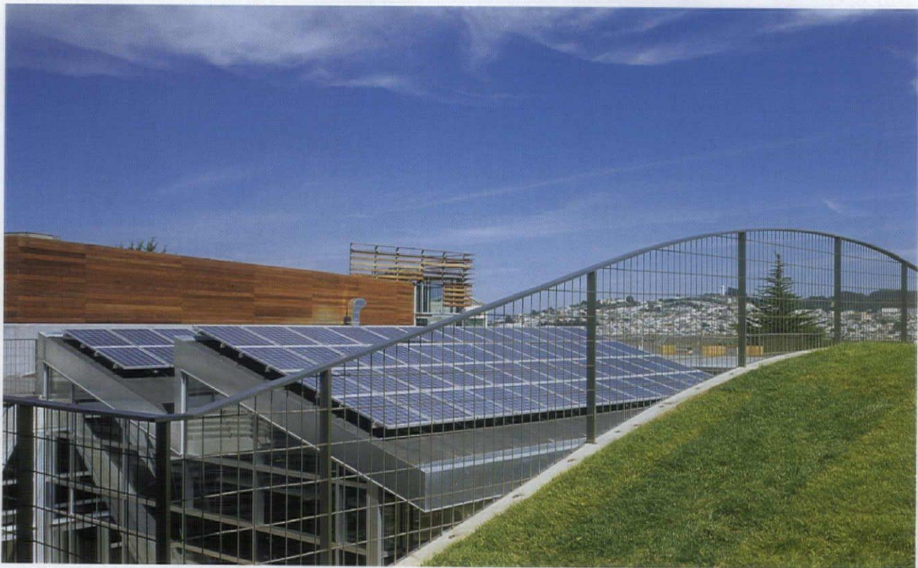
voltaic panels (above). The façade of the double-height cafeteria (facing page) is articulated with a series of louvers placed over the curtain wall. The louvers, constructed of ipé, a sustainable Brazilian wood, reduce heat gain on the structure and introduce a dynamic light pattern on the interior. Behind the shop building sits the theater, also clad in wood, and beyond, the hills of San Francisco.
