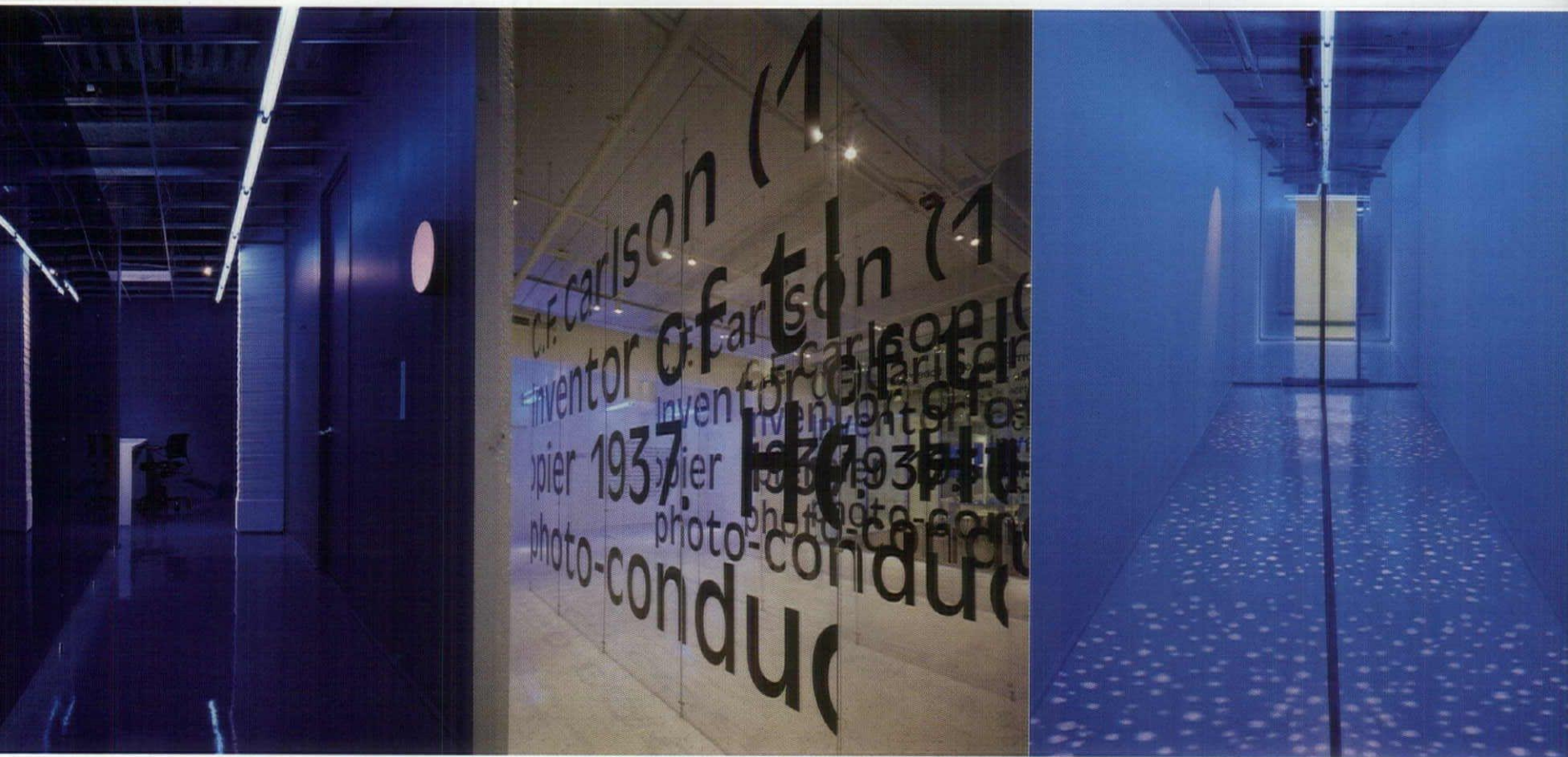
Ceiling-mounted T8 fluorescents with blue tube guards transform a corridor in the Dallas office into a container of blue light. Looking down the hallway toward the reception desk, the left-hand wall, constructed of 1/4-inch-thick transparent blue dichroic acrylic, reflects and amplifies the blue light (above left). In the Oklahoma City headquarters, a series of acrylic word panels line the reception area (above middle). Each office is visually linked to its location. In Washington, D.C., for example, a pattern of cherry blossoms is projected onto the corridor floor. The same hallway aligns with one of the axes of Pierre L'Enfant's original eighteenth-century master plan for the city (above right).
