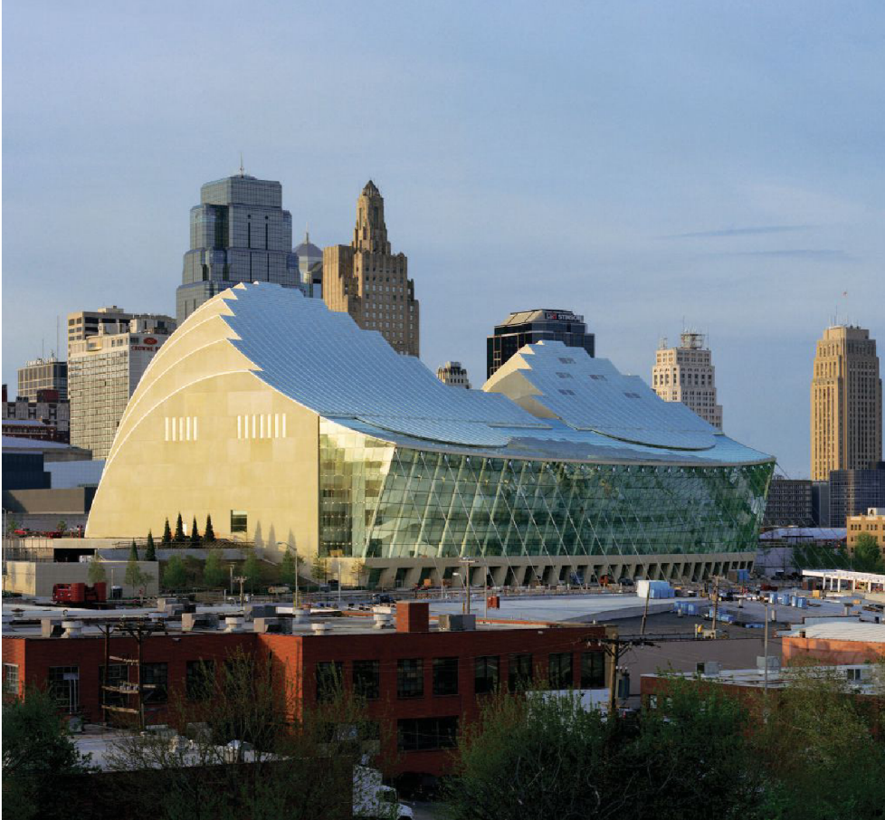
The Kauffman Center's 65-foot-tall by 330-foot-wide glass curtainwall reveals the interiors to passersby (above). The entry drive is anchored by 27 high-tension steel cables (previous page).
