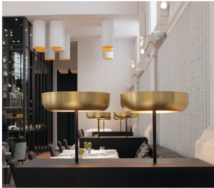
A wall sconce, outfitted with halogen lamps, glass globe shades, and a metal armature is affixed to a brick column outside the wine cellar (far left). Between table areas in the dining room, bronze table lamps using two 25W halogen lamps provide a glow reminiscent of candlelight (left). In the mezzanine bar area (opposite), low-voltage halogen trackheads are affixed to thin, black steel beams that run the width of the space, while maintaining a view to the entire restaurant.
