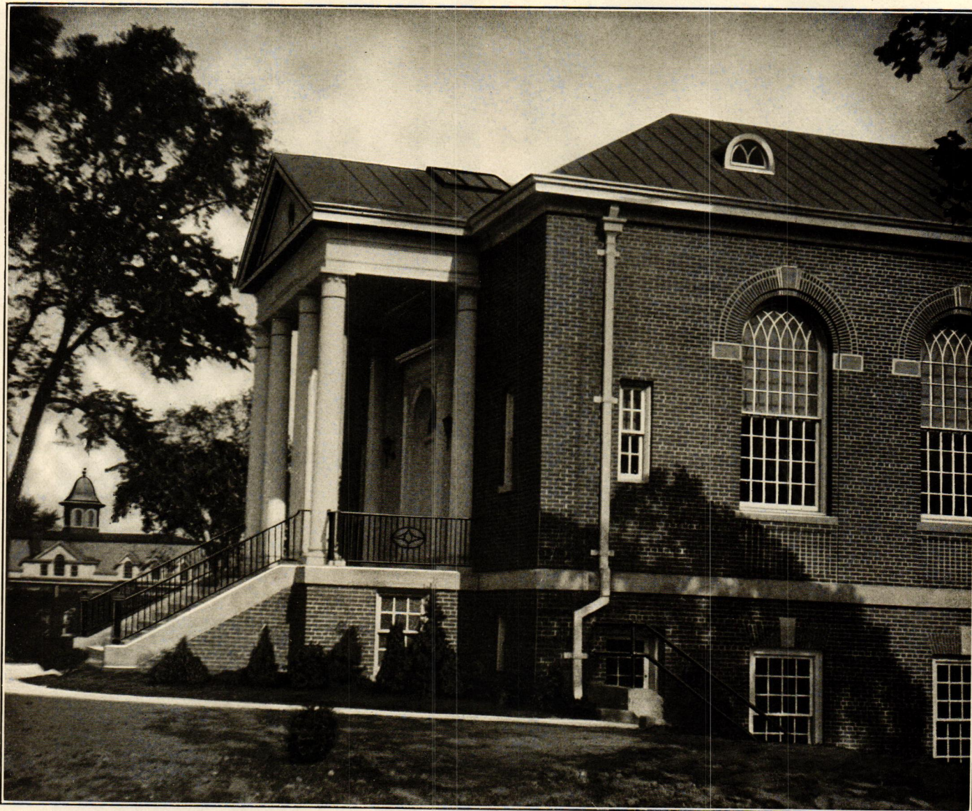
NUTLEY PUBLIC LIBRARY, NUTLEY, N. J. E. J. Mutch, Belleville, N. J., General Contractor
