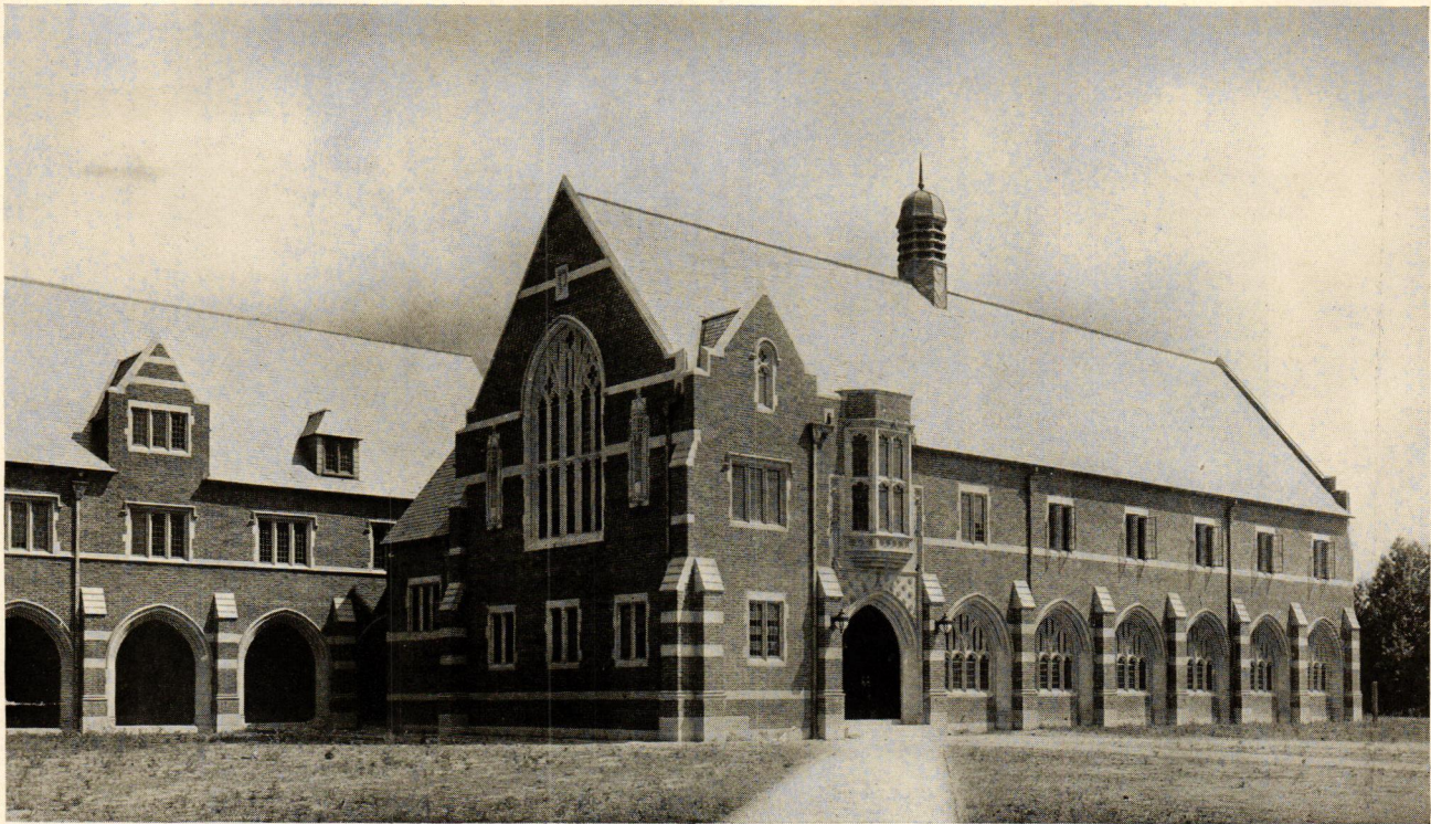
Richmond College Buildings, Richmond, Va., Hydrex-NOVENTO used under all slate roofing Cram, Goodhue & Ferguson and Carneal & Johnston Associate Architects
