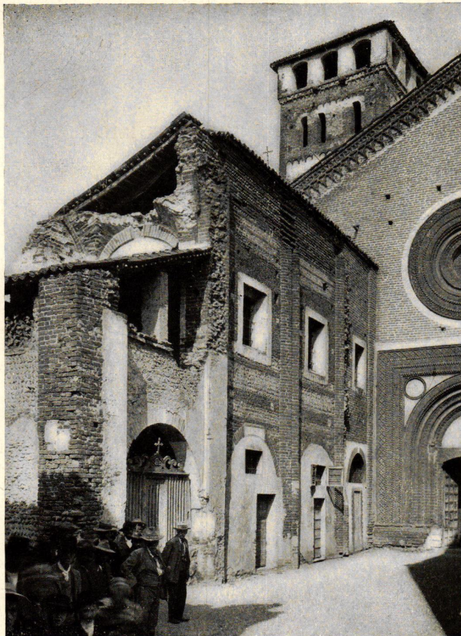
Sannazzaro Sesia. The earliest example of the rib vault (1040).
