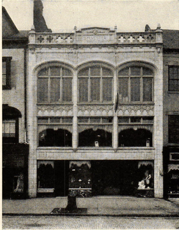
Sylvester Building, Augusta, Ga., G. Lloyd Preacher, Architect. A design of tasteful restraint in granite finish Atlantic Terra Cotta
