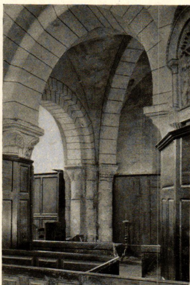
Acy-en-Multien (Oise), probably the earliest rib vault in the Ile-de-France (c. 1100).
