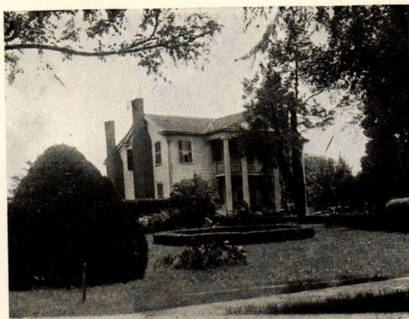
The McCormick Neal Residence, Covington, Ga. The work of a more ambitious amateur showing the Ionic order, yet planned and constructed very simply.
