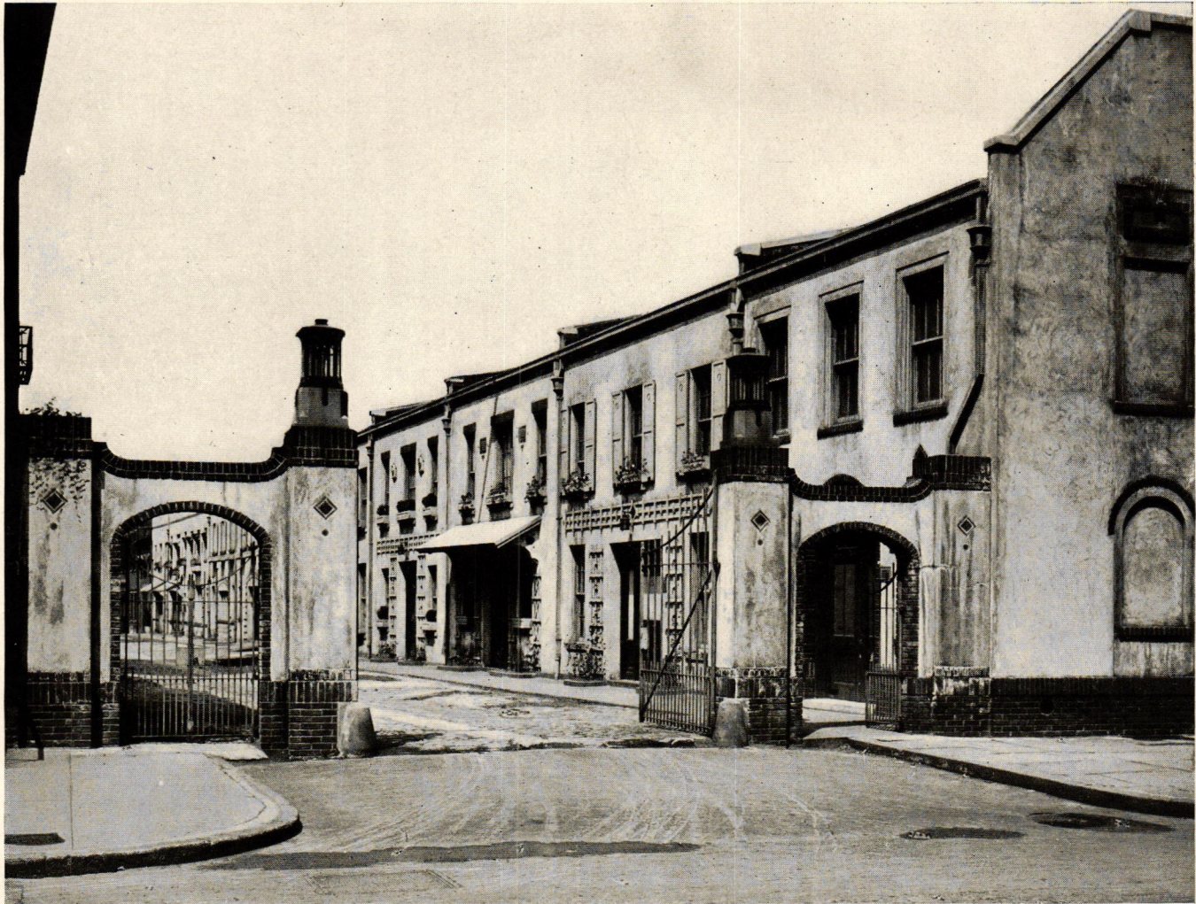
THE WASHINGTON MEWS STUDIOS, ALTERATION OF OLD CITY HOUSES, NEW YORK. Maynicke & Franke, Architects. Honorable mention A. I. A., 1917.
